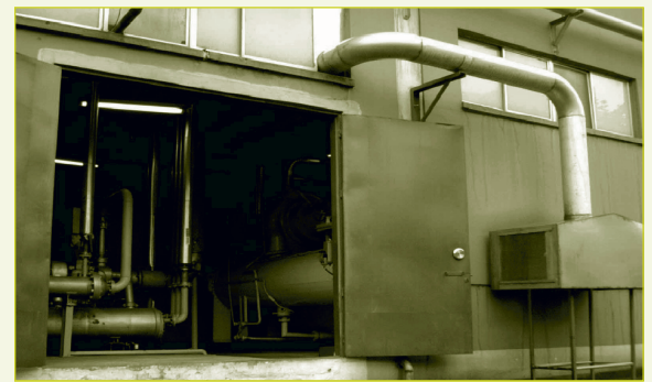
Air compressor—air inlet relocated to outside compressor room
